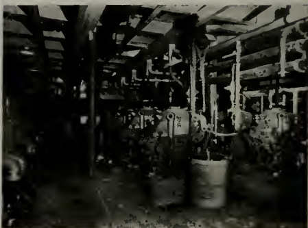
View of the Separator Room.
